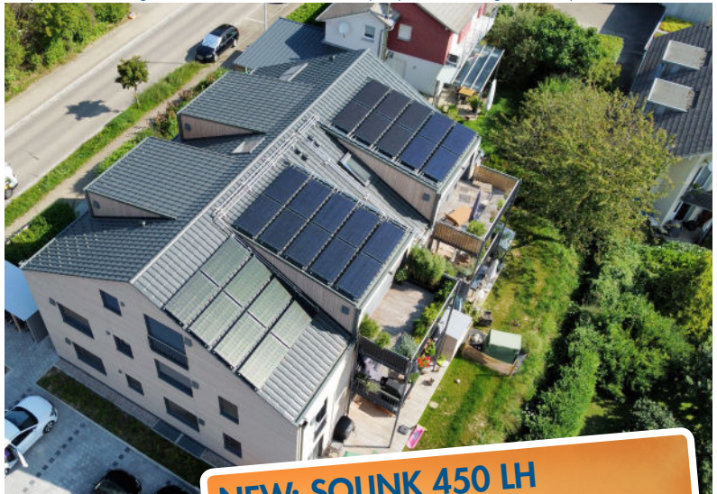
Apartment building with 6 flats and a 17 kW heat pump near Freiburg, Germany
